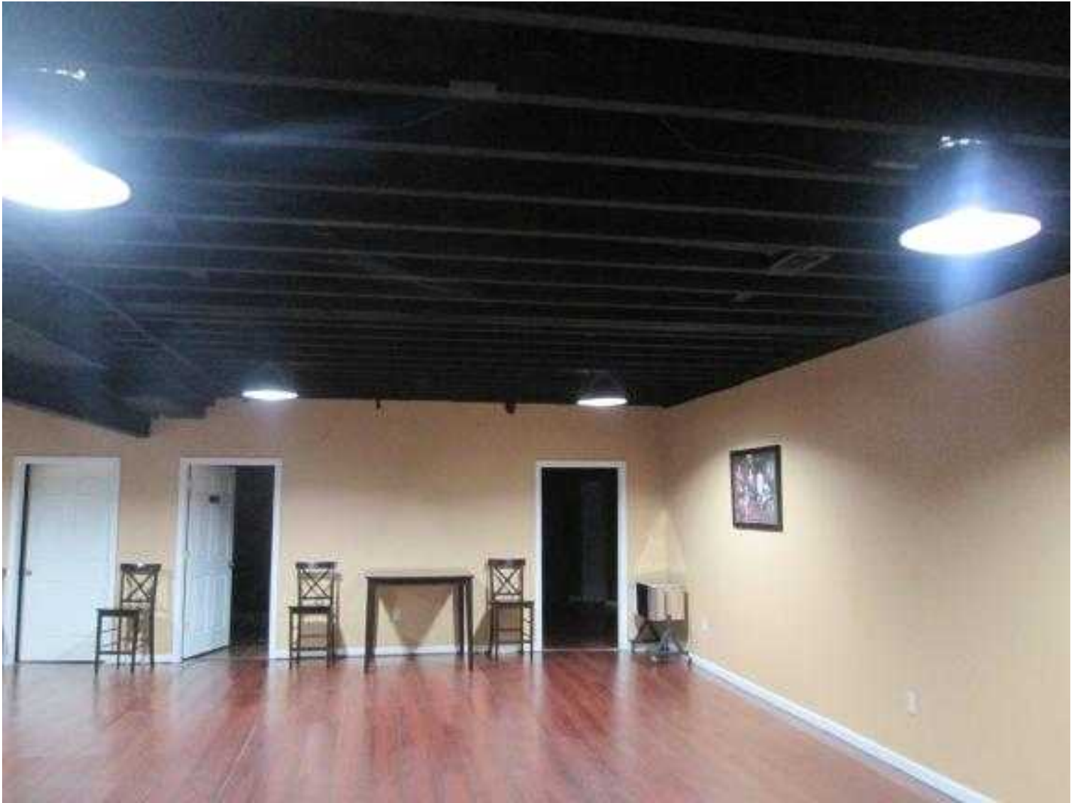
#44 laminate floor, bad idea. It will absorb moisture through the concrete floor and swell then buckle.
