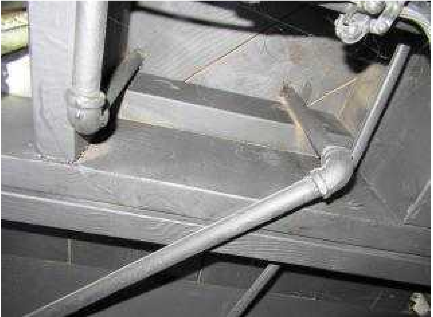
#40 Close up of what the pipes and structure look like once painted.
